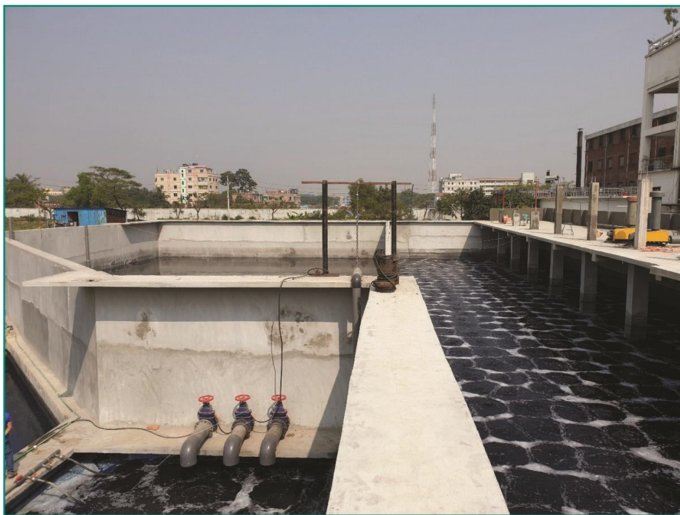
Fig. 4: The New 11,890 m 3 Equalization Tank
