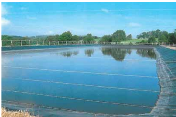
Fig. 3: The second lagoon was completely cleared of solids after the six-month PIT PERFECT® pit treatment.
